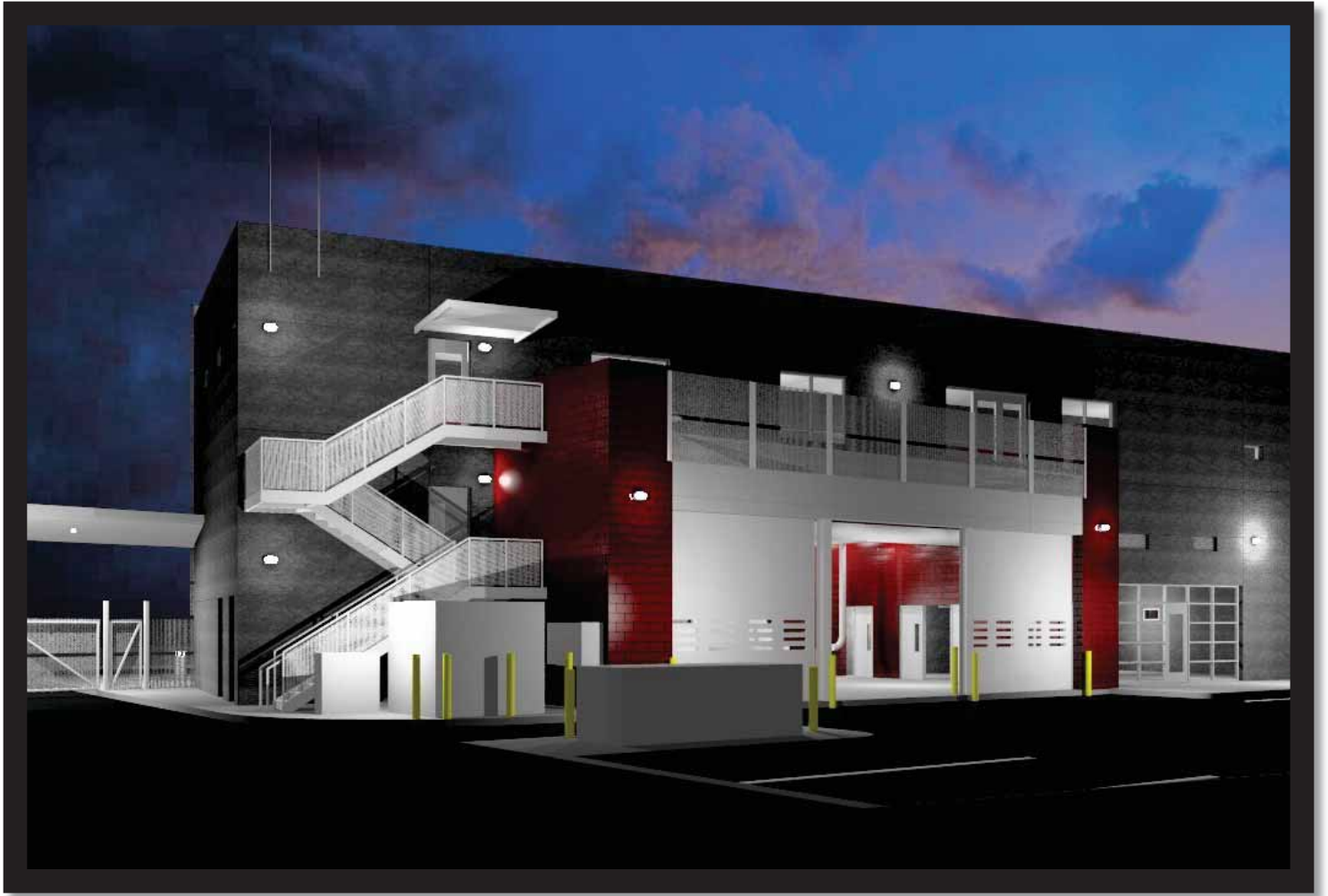
Farmington Fire Station #1 Remodel
