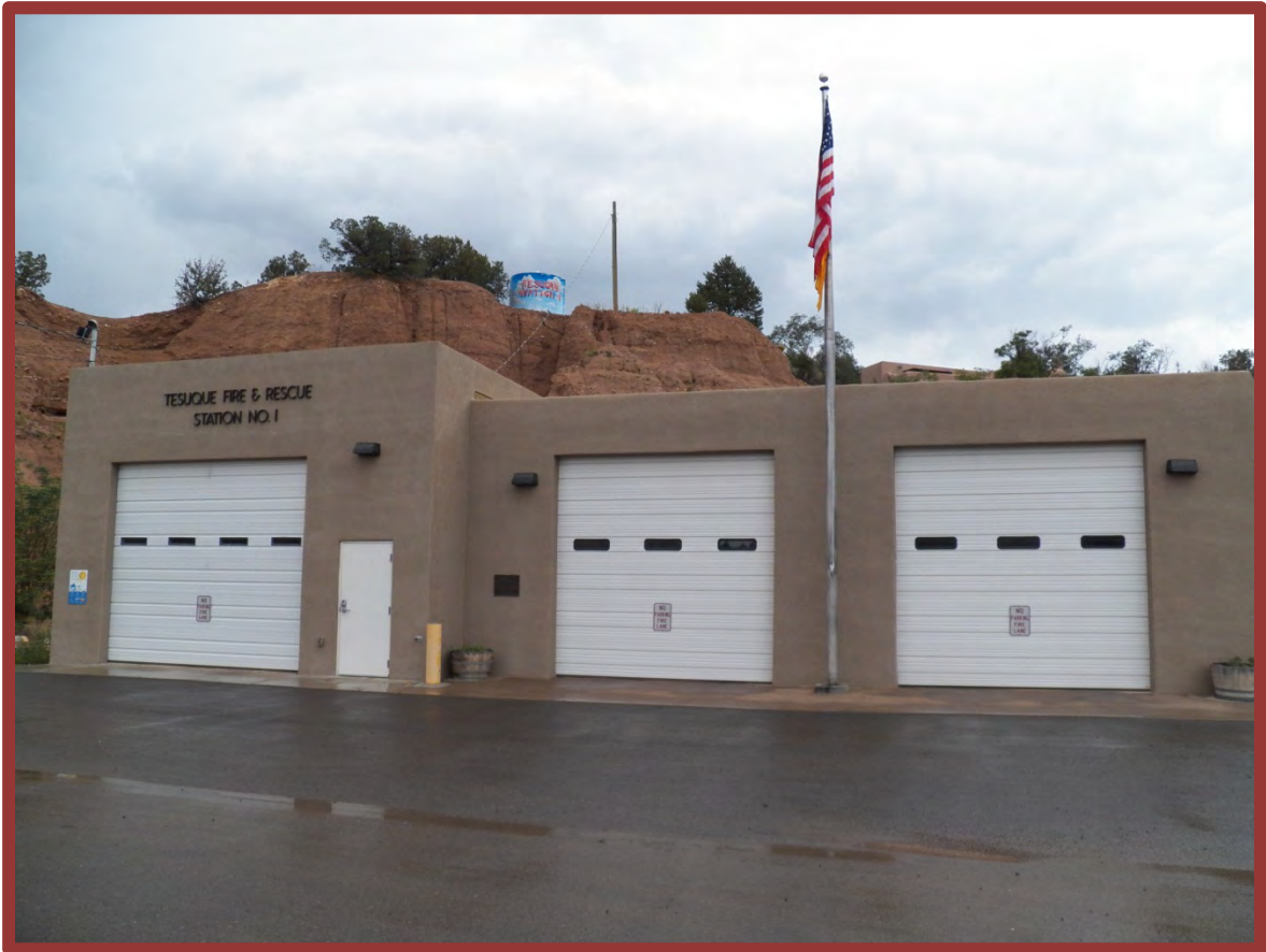
Tesuque Fire Station
