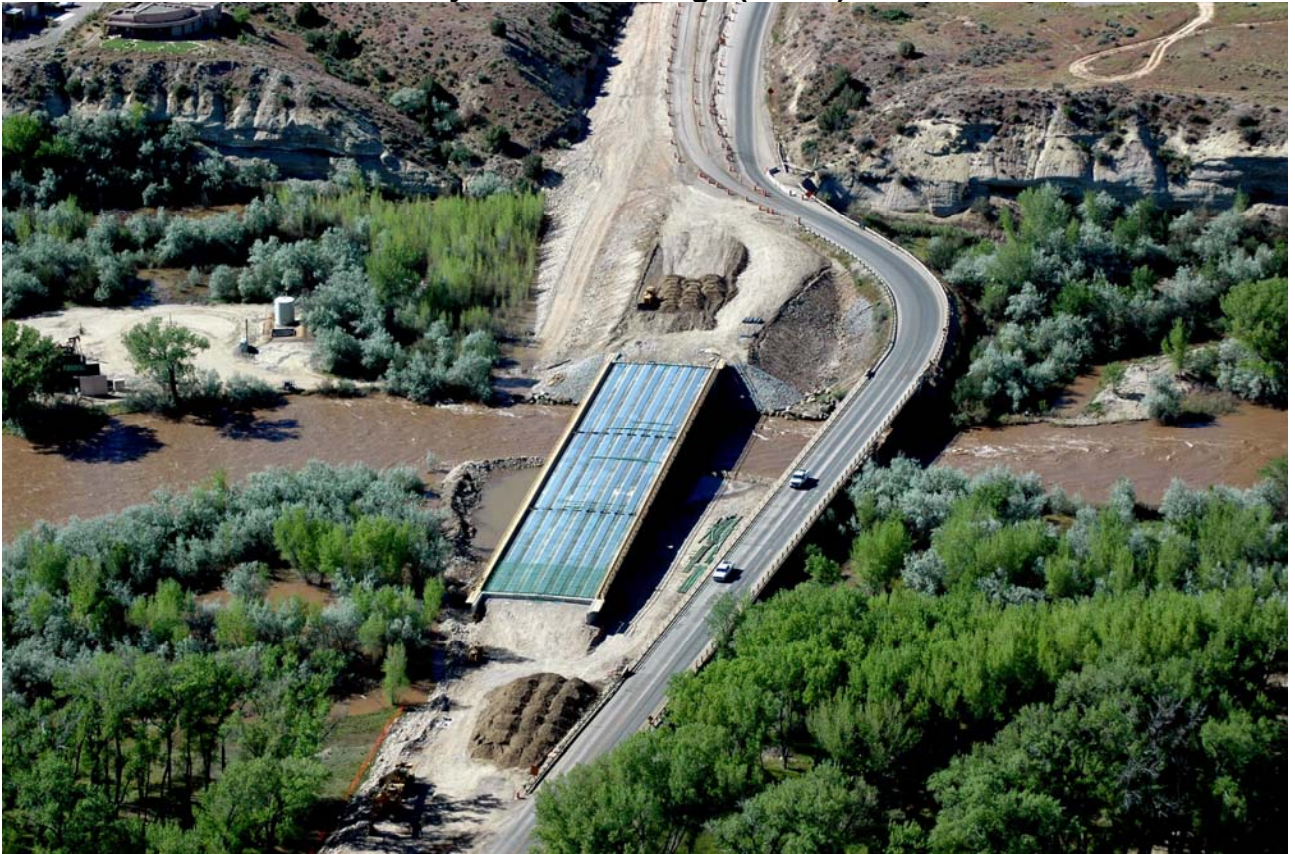
County Road 350 Bridge (Aerial)
