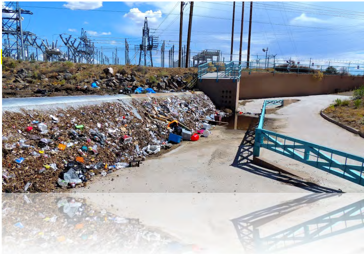
Water Quality Structure, before and after a storm, captures debris before it reaches the river
