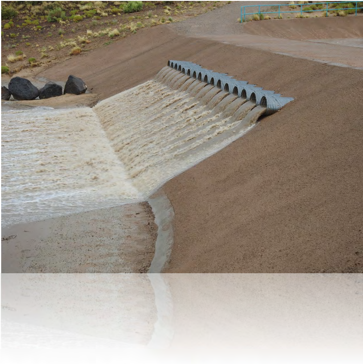
Black Arroyo Dam Water Quality Structure during summer monsoon
