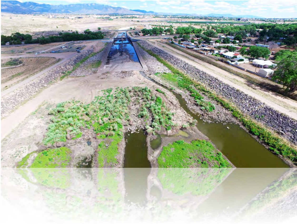
Settling basin for the North Diversion Channel
