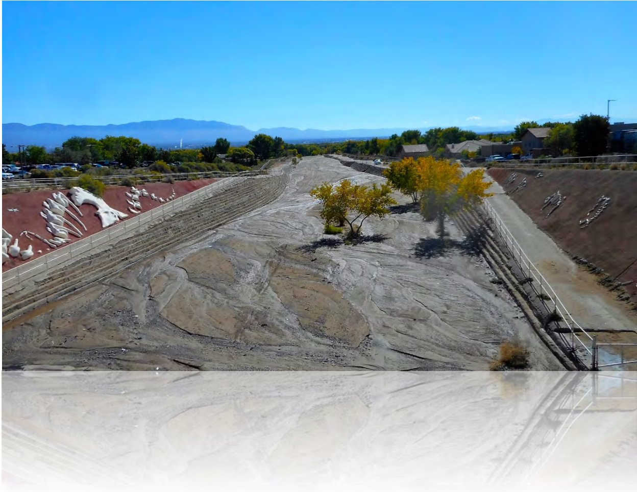
Calabacillas Arroyo at Coors Road, Northwest Albuquerque, 1998 improvements
