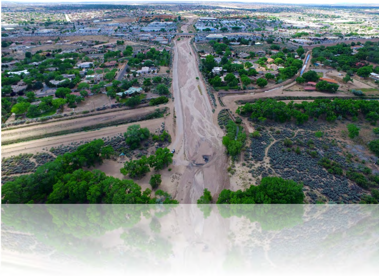
Outfall for the Calabacillas Arroyo
