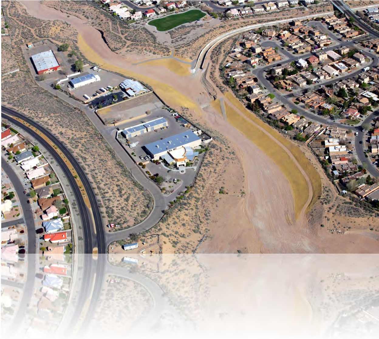
An aerial view of the Calabacillas Arroyo, including the recently constructed Grade Control Structure 6a
