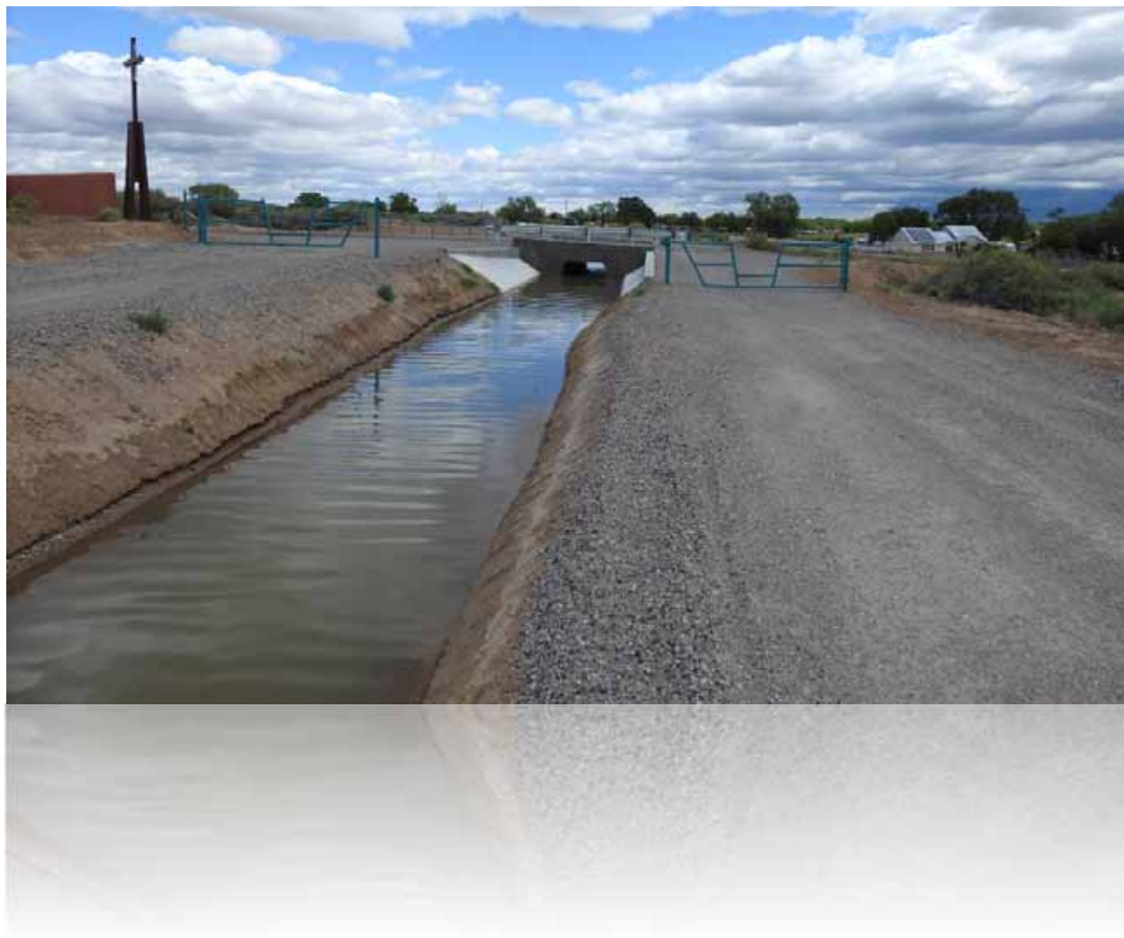
Before and after views of the Black Mesa Facility's Dominican Crossing
