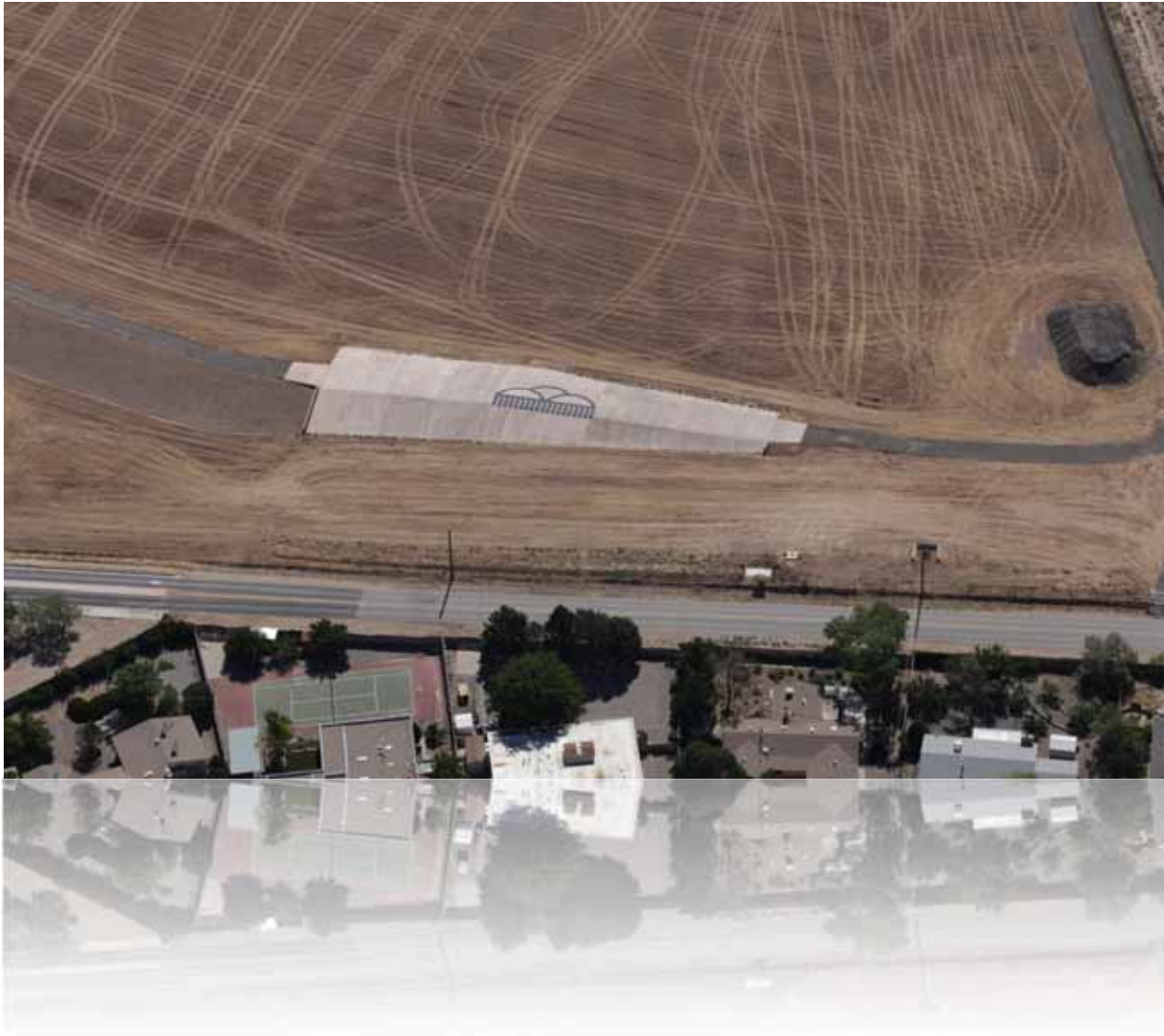
The new spillway at Louisiana & Gibson has a familiar look
