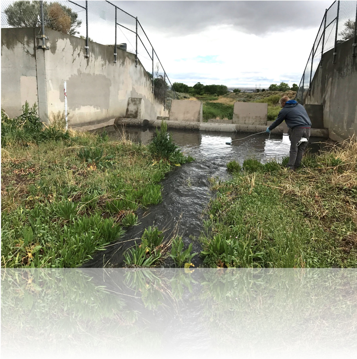
Energy dissipation structure on the Bear Canyon Arroyo
