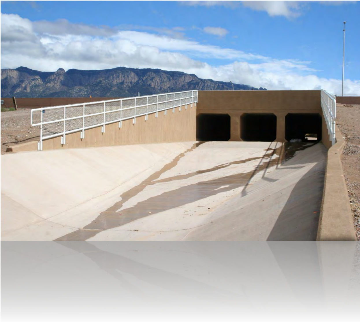
North Camino Arroyo Crossing at I-25
