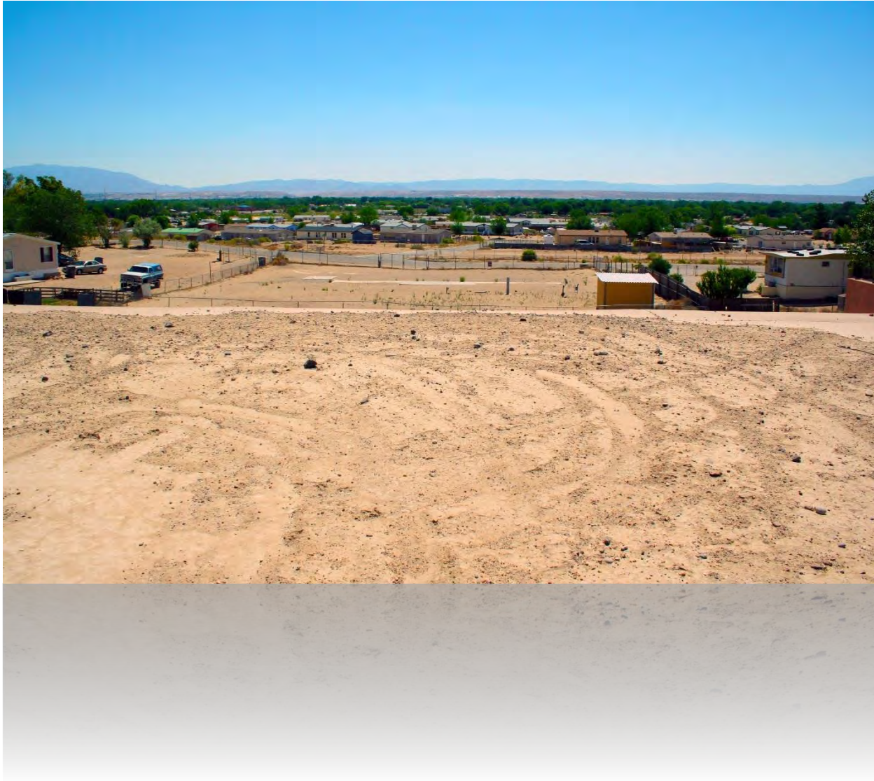
Don Felipe Dam, located on the Albuquerque's Southwest Mesa, protects portions of the southwest valley from flooding
