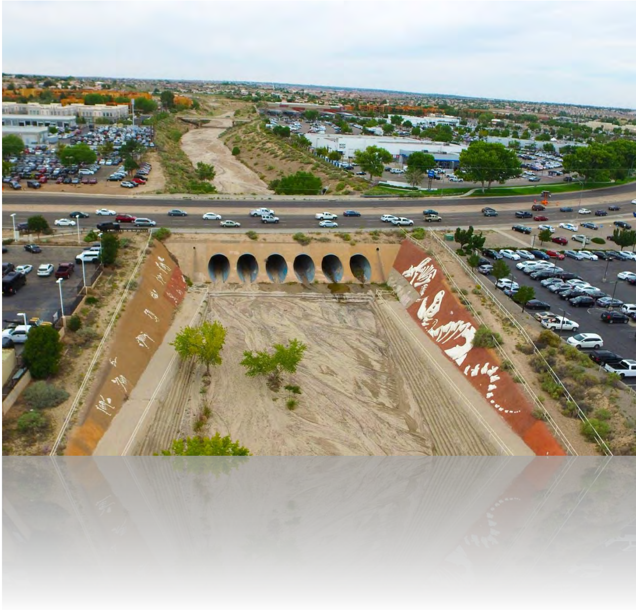
Calabacillas Arroyo at Coors Road, Northwest Albuquerque, 1998 improvements
