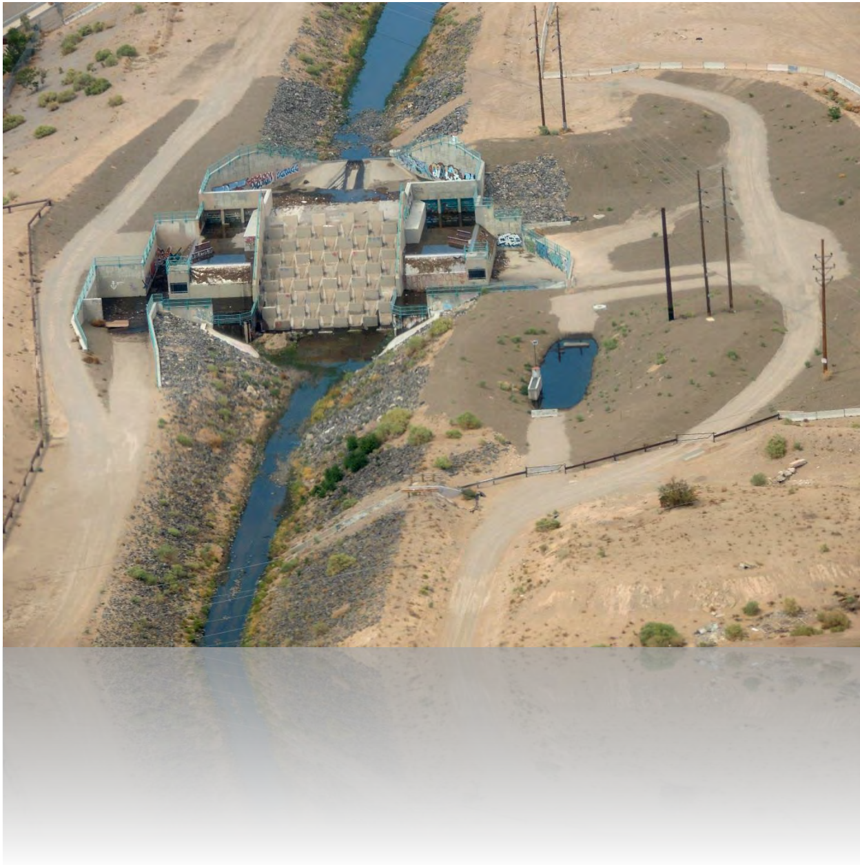
South Diversion Channel, Baffle Chute Water Quality Structure, constructed in 2011
